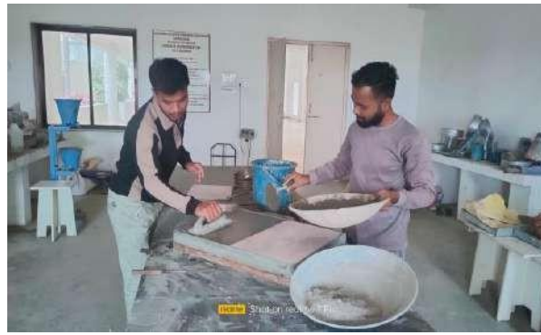
figure b- preparing surface for epoxy resin flooring
